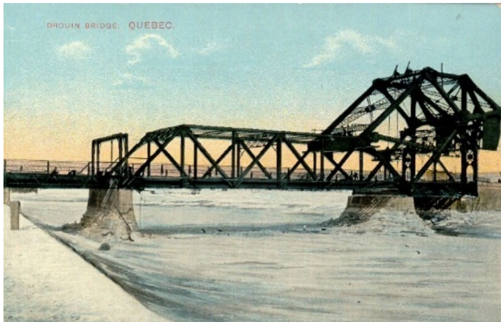
Figure 51 « Drouin bridge. Quebec » (BAnQ P547S1SS1SSS1D001P0391R)
